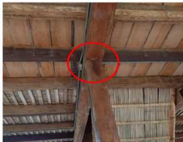
ENSAMBLE CAJA Y ESPIGA USADO EN UNIONES ENTRE COLUMNA Y VIGA.
